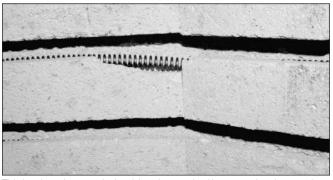
This is minor damage. It should not be repaired because the element does not bulge outside the groove; the brick still supports the element. Also, the groove does not insulate the kiln. The part of the firebrick that insulates is between the kiln's outer steel case and the elements.
