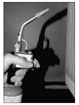
After you have cemented the brick patch, heat the cement seam with a propane
