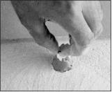
into the hole until the plug is flush. Wipe off excess cement. If necessary, sand after the cement has dried.
