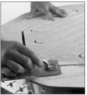
If you are coating over a freshly patched firebrick surface, allow the cemented patch to dry first. **Liquid Kiln Coating Instructions**
